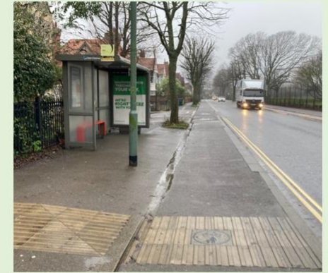
Bus stop boarder, stepped track cycle lane and removal of centre lines (Old Shoreham Road, Hove)
