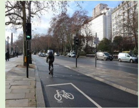
Fully separated cycle lanes (bi-directional), Embankment, London
